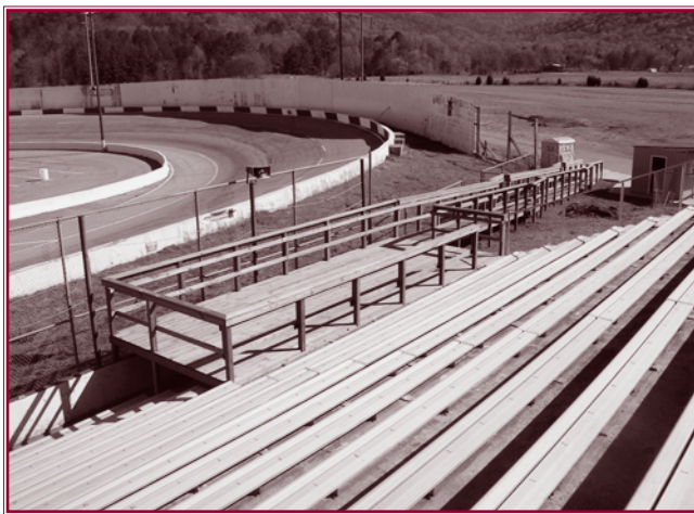
A ramp and accessible seating at the Huntsville Speedway in Huntsville, Alabama.
